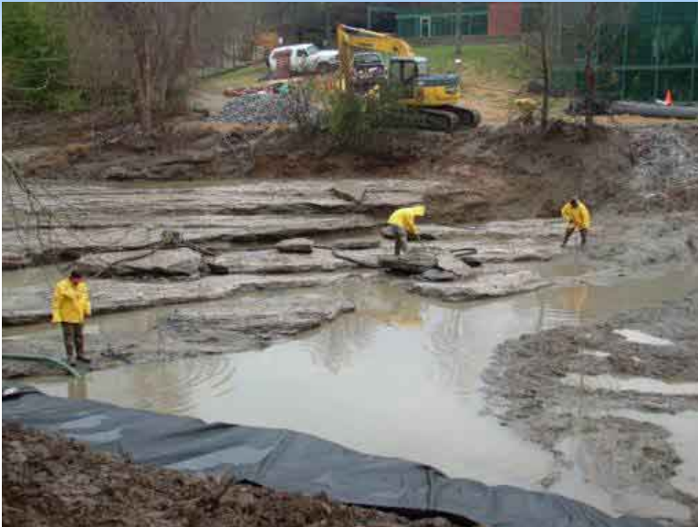
Pumping off of excess water to expose the sediment before removal.
